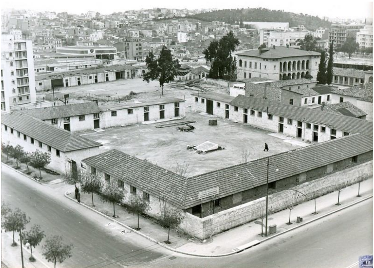
The Artillery barracks in which the National Gallery was housed.
