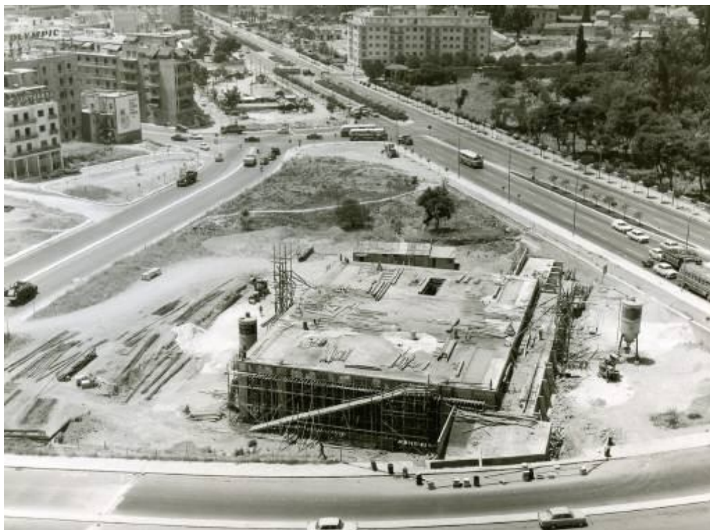
A section of the National Gallery building during construction
