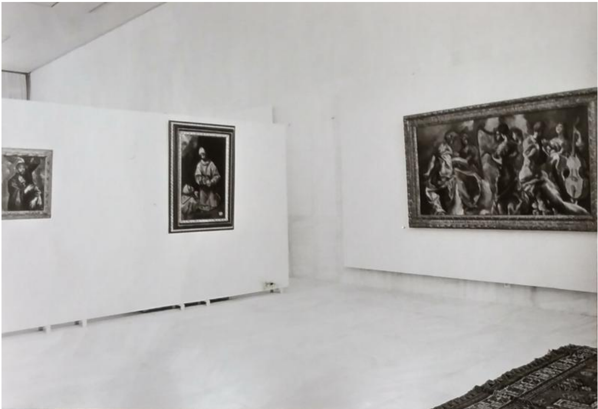
Section of the exhibition dedicated to Domenikos Theotokopoulos (El Greco) at the inauguration of the first building in 1970
