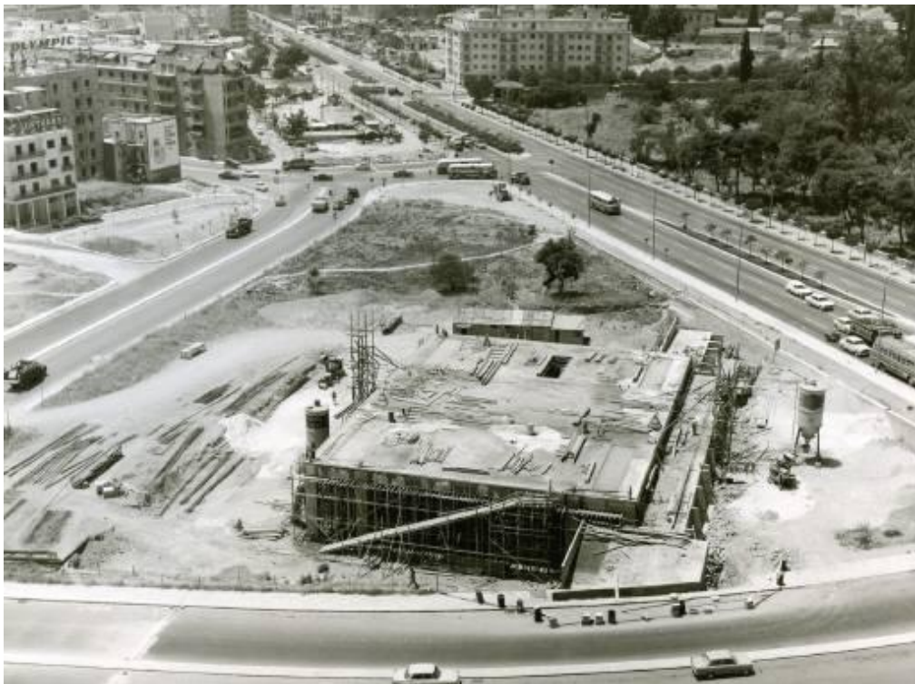
First section of the National Gallery building during construction
